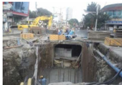
Mandaluyong Main Drainage Project
