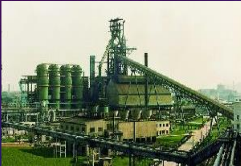
Example of a Chinese blast furnace used for smelting limonite nickel ore,
