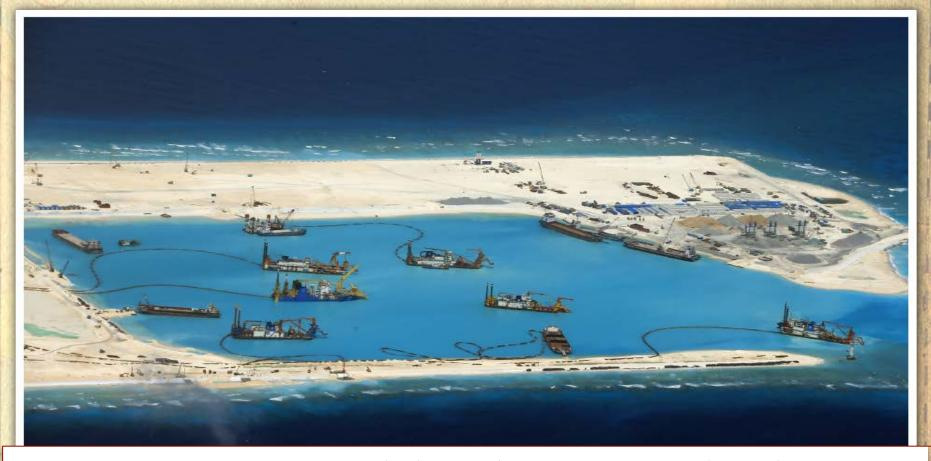
Seven (7) cutter suction dredgers and seven (7) cargo/supply vessels at Kagitingan (Fiery Cross Reef
