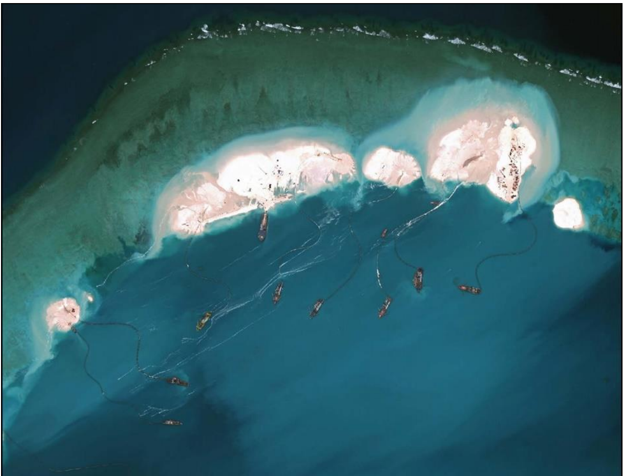
Figure 17: Dredgers at work at Mischief Reef (Annex 792)
