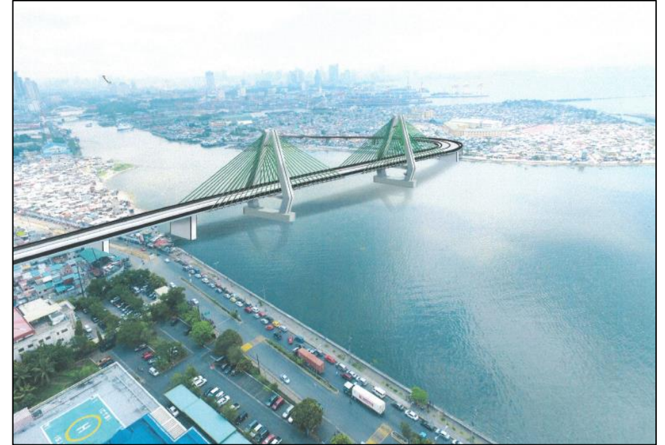
Future bridge adjacent to MICT
